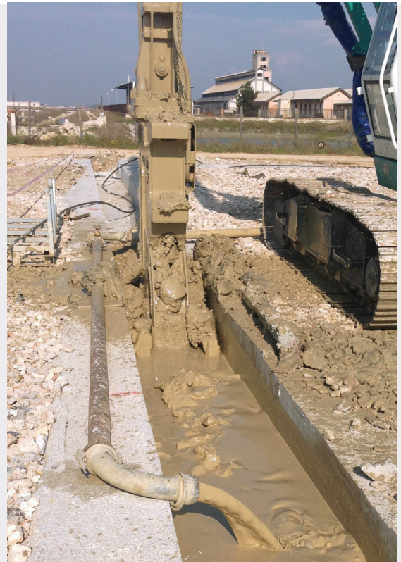
60-cm barrier. Barriers up to 1.2 m wide can be built
