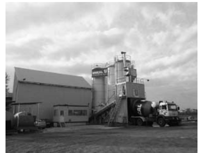
Ready-mix batch plant
