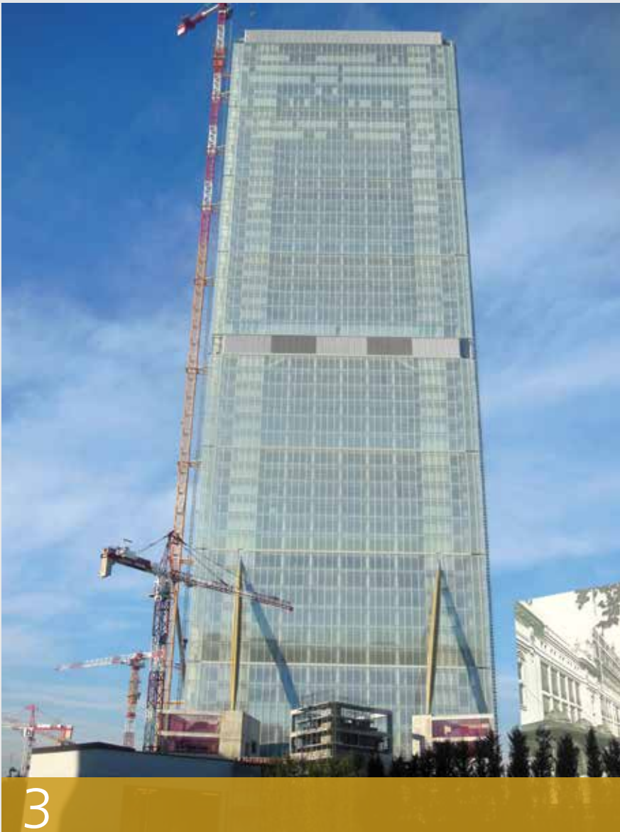
3. TORRE ISOZAKI - STRUTTURA ULTIMATA NOVEMBRE 2014 / ISOZAKI TOWER – COMPLETED IN NOVEMBER 2014
